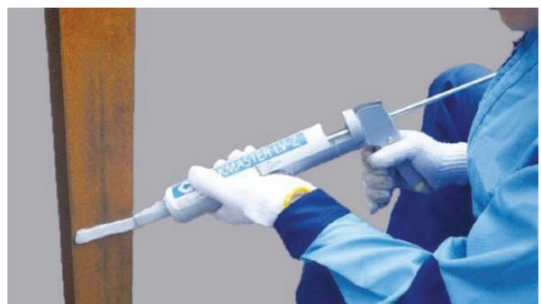
5. Apply Leakmaster continuously without a break to the place to be sealed.
