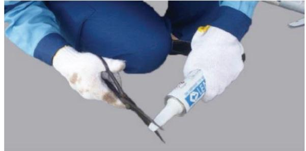
2. Cut the nozzle at the appropriate position diagonally.
